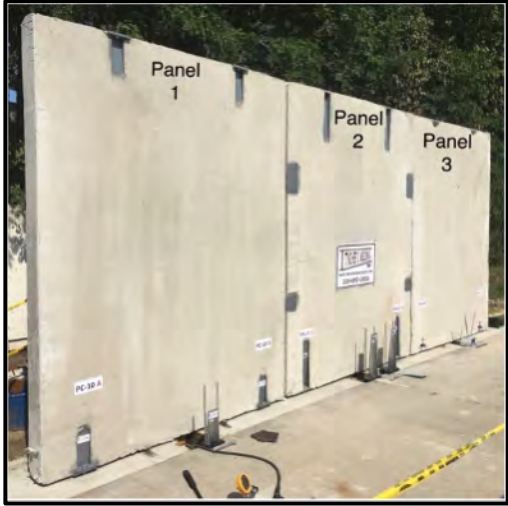
(a) Panels before bracing
