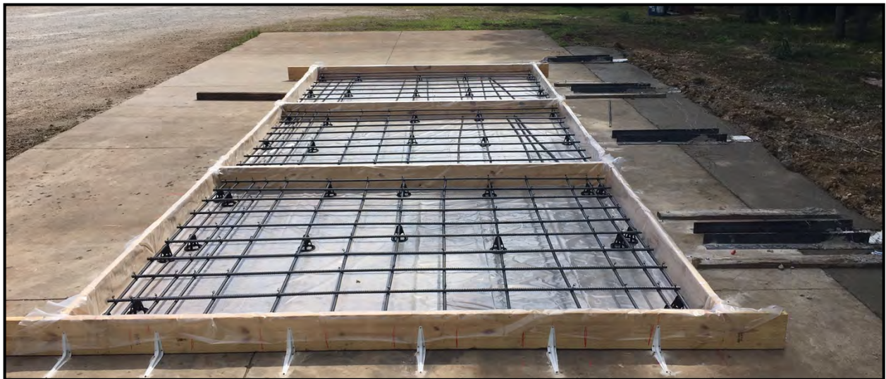
(b) Panels before concrete placement
