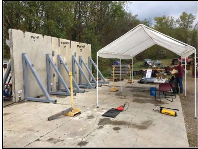
(b) Panels after installation of lateral braces
