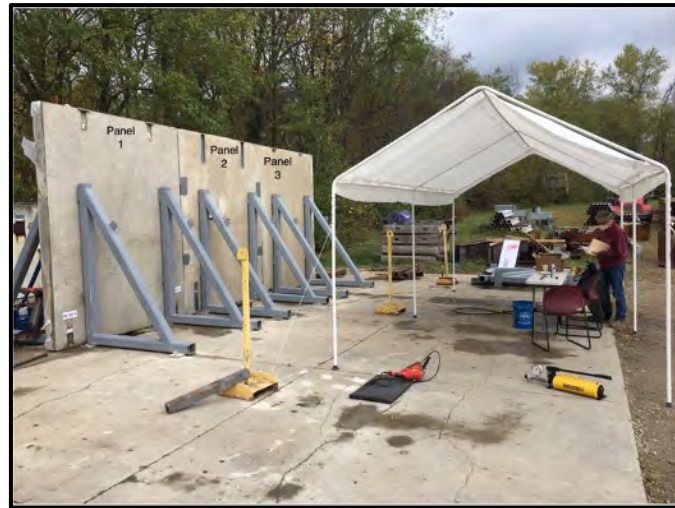
(b) Panels after installation of lateral braces
