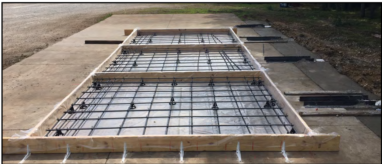
(b) Panels before concrete placement
