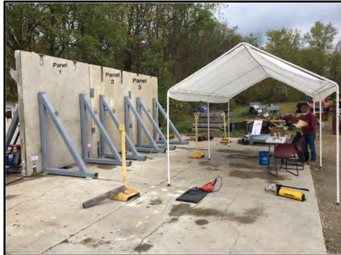
(b) Panels after installation of lateral braces
